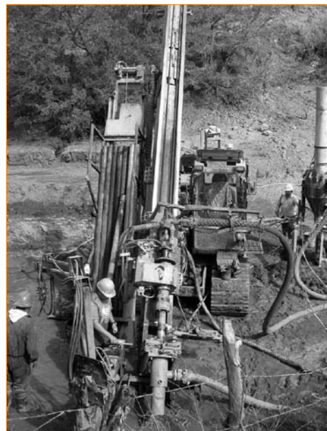
RC resource definition drilling at El Rayo
